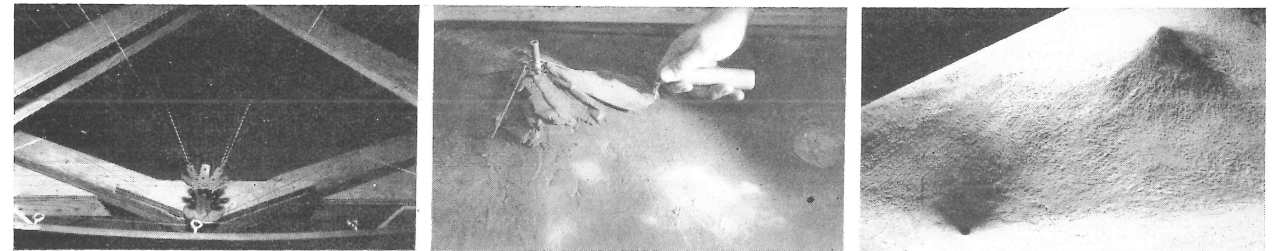
37. Stretching the metal net. 38. Finishing the concrete at summits. 39. Finished summits and low vertex of the square perimeter model, surface was finished with brush.
