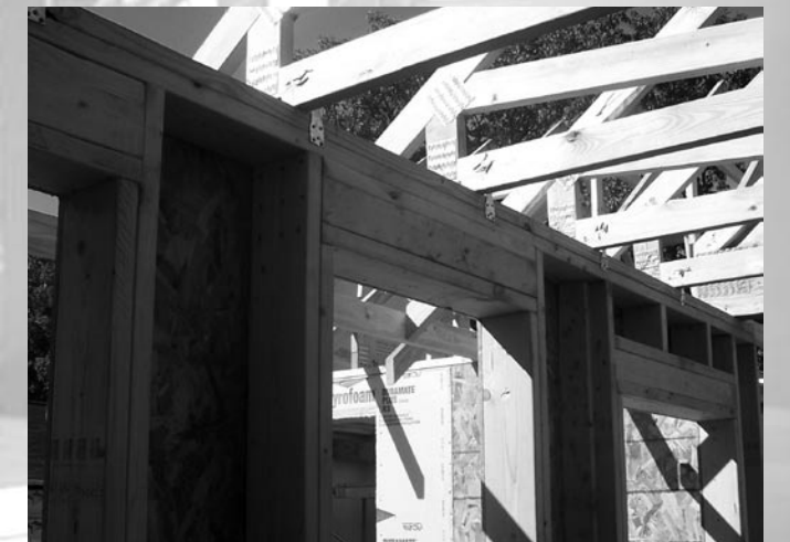
Building detail of the Hillsborough home in Orange County during construction including advanced in-line framing and raised-heel energy trusses.
