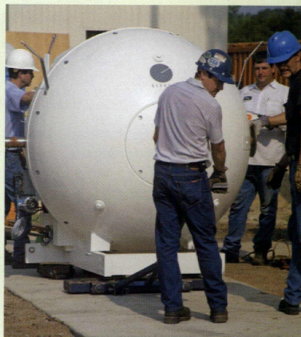
It's moving day for a new Gamma Knife at Pitt County Memorial Hospital. Its housing is five feet in diameter and weighs 20 tons
