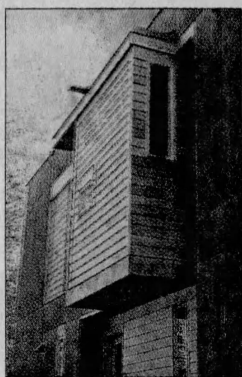
The lapped cedar boards add detail and texture to the exterior walls of the 2,500-square-foot home.
