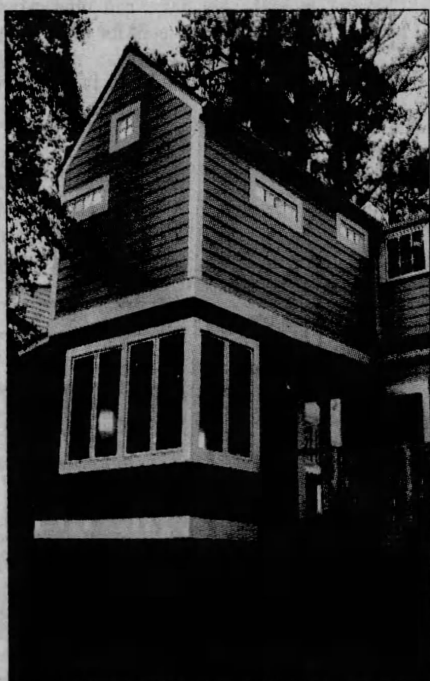
For the large openings that connect the addition to the backyard, Hardi-panels were used instead of the wood siding on the existing part of the house.
