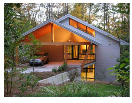
The house sits a few feet below the elevation of the street, allowing its simple gabled roof to rise no higher than its neighbors. The footprint of the house - a simple 32-foot-by-54-foot rectangle - draws its dimensions from the 1960s-era ranch-style house next door. A covered carport, rather than a garage, gives depth to the street view.
