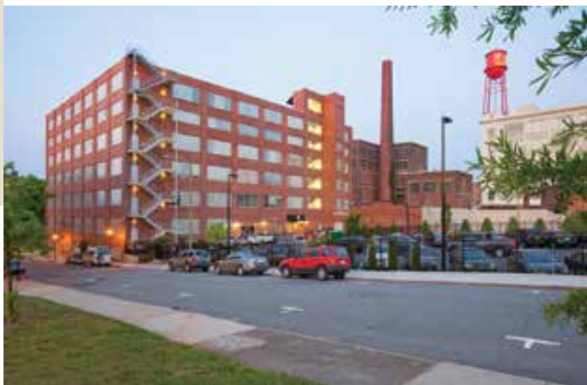
The Hanes Knitting Company Warehouse building after rehabilitation was completed.
