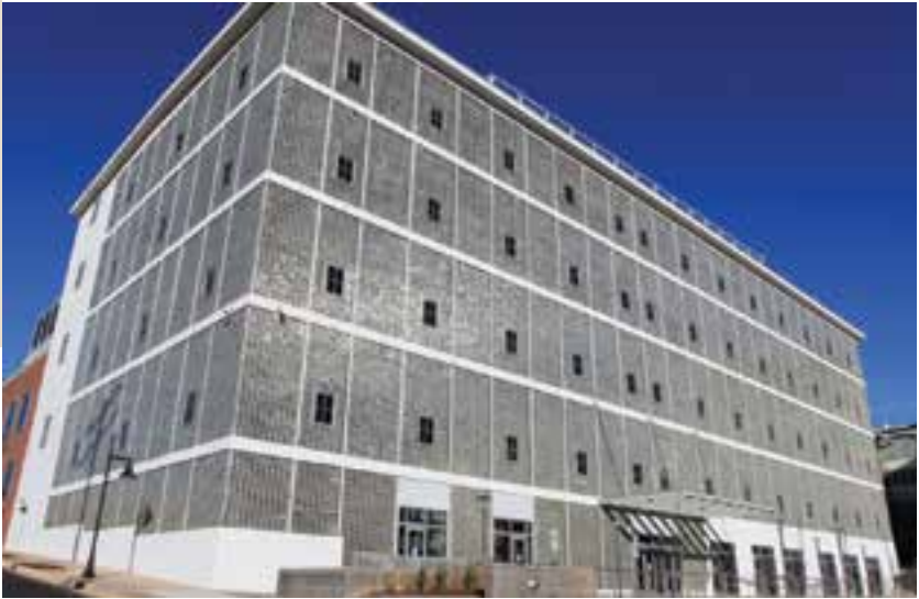
The former RJ Reynolds Factory 91 in Winston-Salem after rehabilitation. Right, the 2012 grand opening ceremony for the new Wake Forest BioTech Place.
