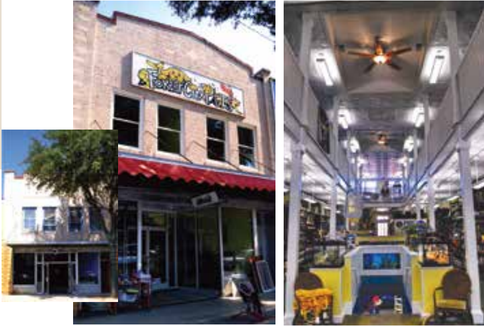
Forest City Pets Store, before (inset) and after. On the right, the multi-level interior of the pet store with pressed-tin ceilings.
