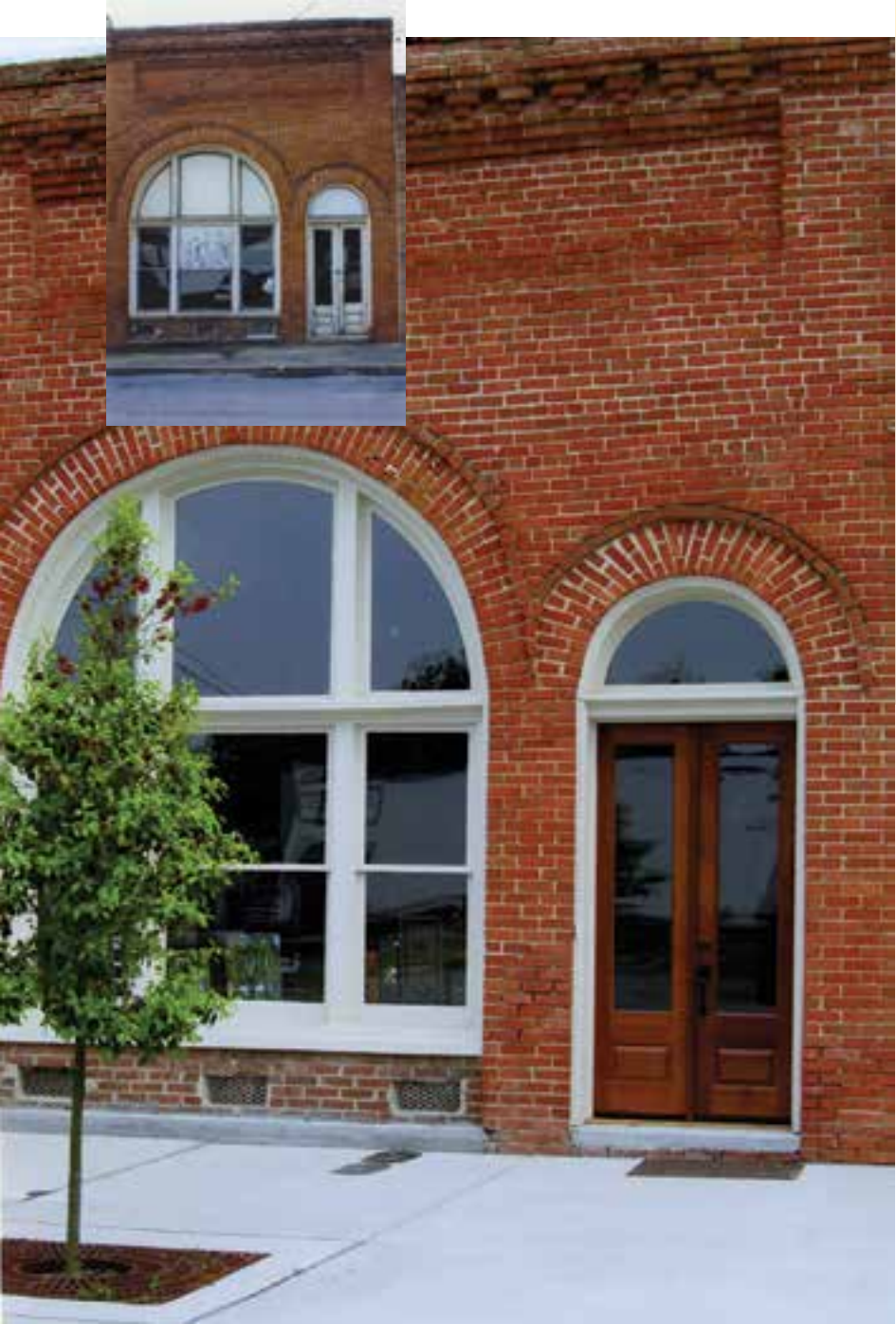
The Bank of Four Oaks building in Four Oaks, before (inset) and after.
