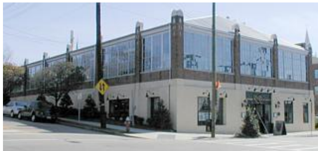
116 North West Street
