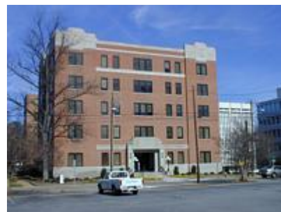
Caswell Office Building
