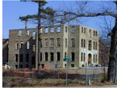
St. Augustine's College (St. Agnes Hall renovation)
