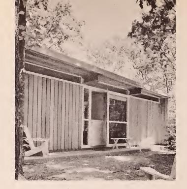
prefabricated price which would have provided none of the amenities and would have had only about 75% of the floor area. The exposed framework leaves spaces which provide handy shelves, used to advantage primarily in the kitchen, bedrooms and bathroom. The house plan is as simple and direct as the construction system.
