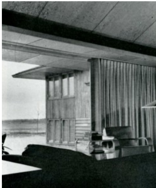
Sun control is handled by broad roof projections.
