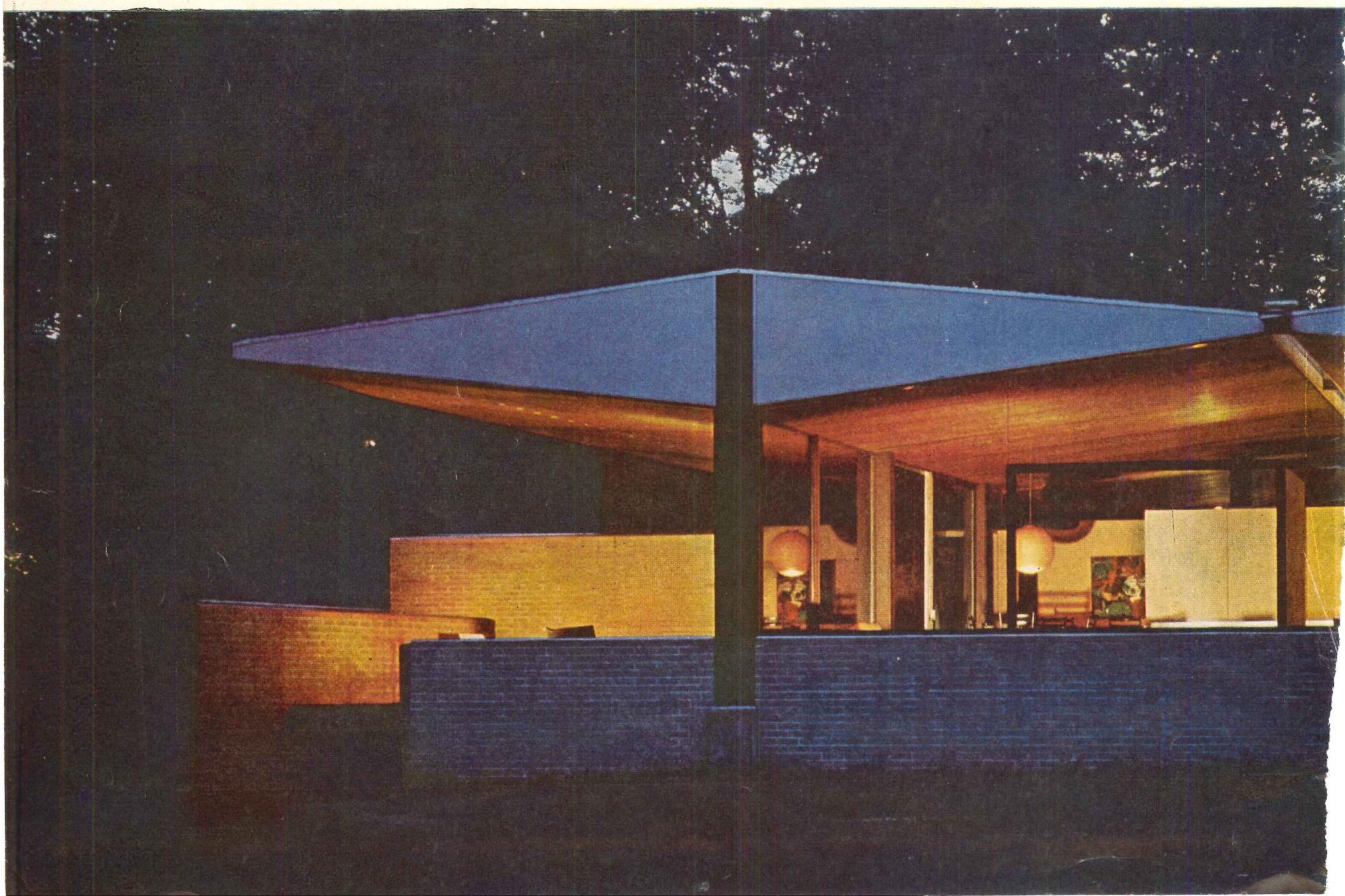
BATWING HOUSE in Raleigh, N.C. was built in 1955 by Argentinian Eduardo Catalano. It is essentially a six-room glass box roofed over by a giant 3,600-square-foot geometric form known as a hyperbolic paraboloid. Its doubly curved
