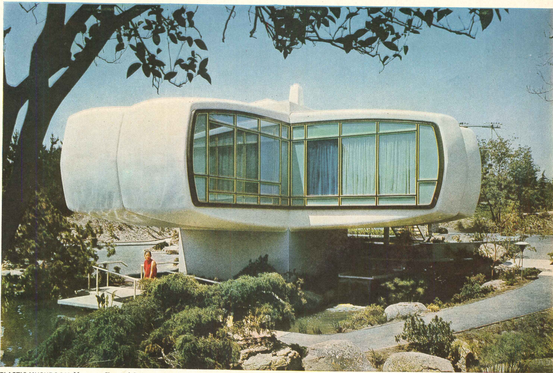
PLASTIC MUSHROOM , Monsanto Chemical Co.'s experimental house, consists of only 20 molded pieces. Whole house rests on a 16-foot-square block of concrete. The four wings are cantilevered from utility core in center. Floors and
