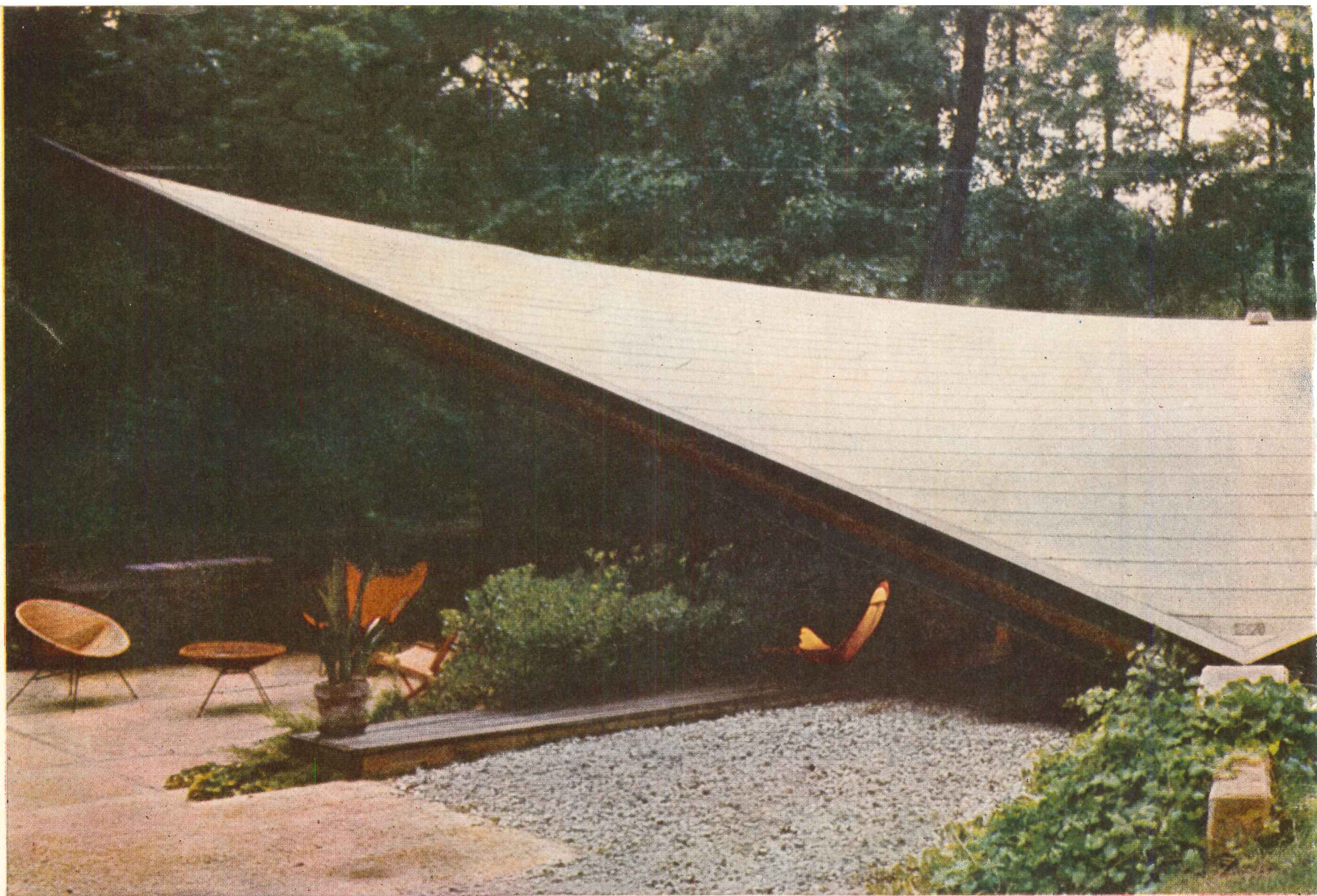
BATWING HOUSE in Raleigh, N.C. was built in 1955 by Argentinian Eduardo Catalano. It is essentially a six-room glass box roofed over by a giant 3,600-square-foot geometric form known as a hyperbolic paraboloid. Its doubly curved
