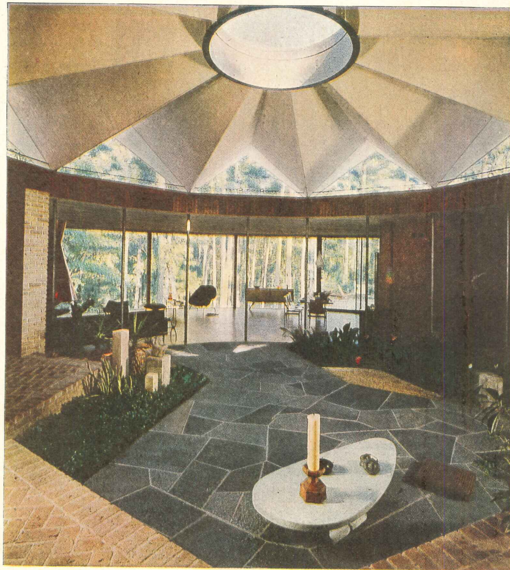
CREASED ROOF , on a house in Atlanta, is made of laminated plywood folded around plastic skylight and held together by cable threaded through lower edge. Light and cheap, it provides unsupported span for modern, uncluttered interior.
