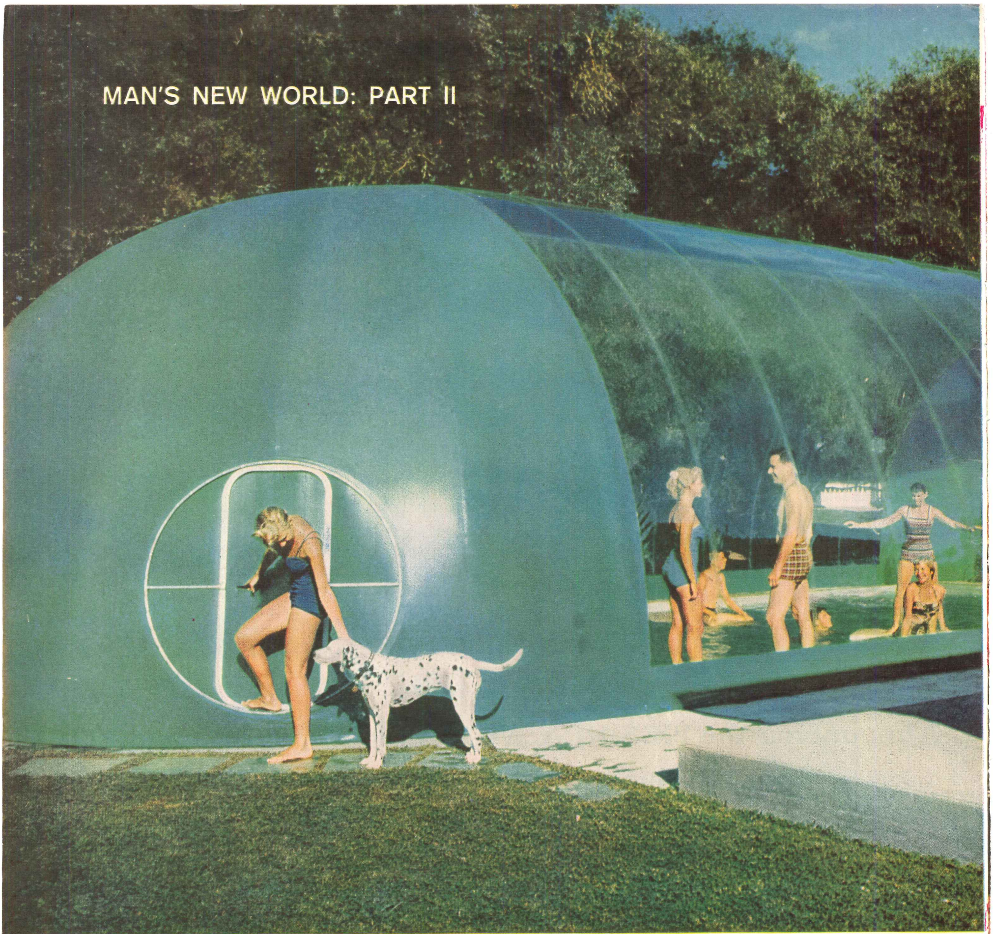
PLASTIC COVER, BLOWN UP LIKE A BALLOON, SHELTERS SWIMMING POOL IN BACKYARD OF BUFFALO INVENTOR WALTER BIRD SUMMER AND WINTER. AIR BLOWER
