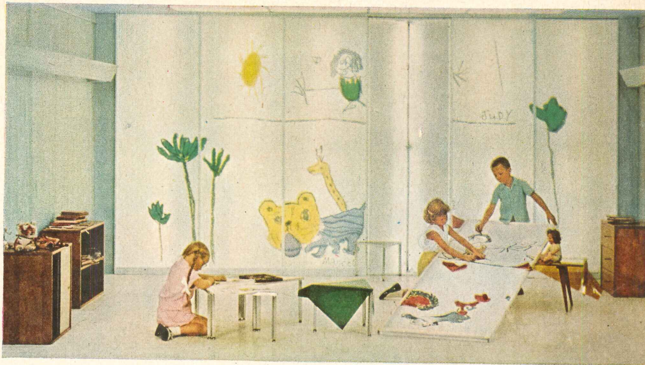
LUMINOUS WALL , by General Electric, consists of translucent Fiberglas panels covering 60 four-foot fluorescent tubes. In the child's room above,
