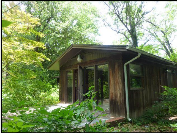
Upper slate patio
